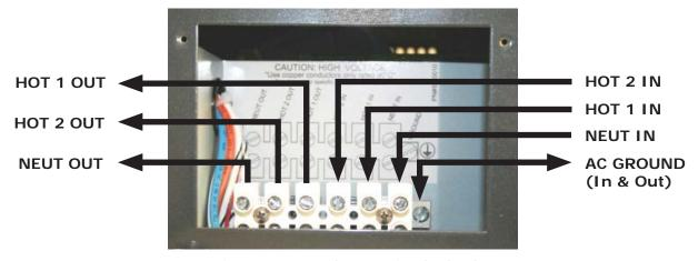
Figure 2-9, AC Terminal Block
