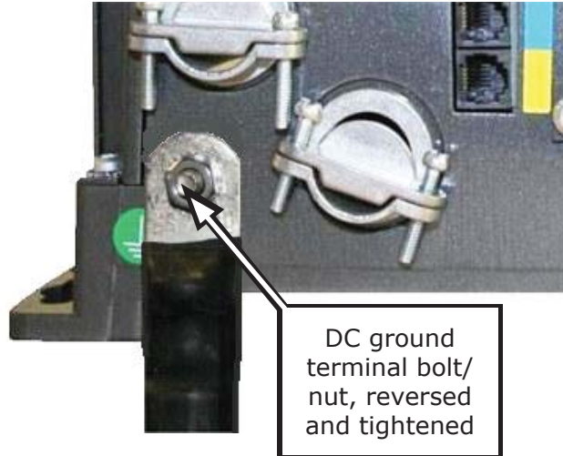
Figure 2-15, Connecting a Large DC Ground Wire
