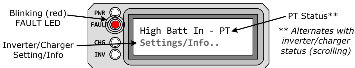
Figure 10-9, PT Controller Fault Message (Example)
